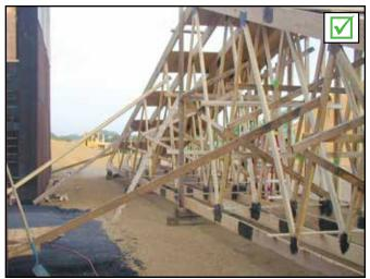
Ground Bracing for Truss assembly being built on the ground. **PHOTO B2-9**
